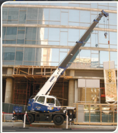
15 ton Tadano used for its compact size on 1400 S. Michigan.
