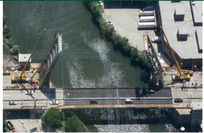
**Based on engineering of the bridge it has to be in the upright position to dismantle.**
