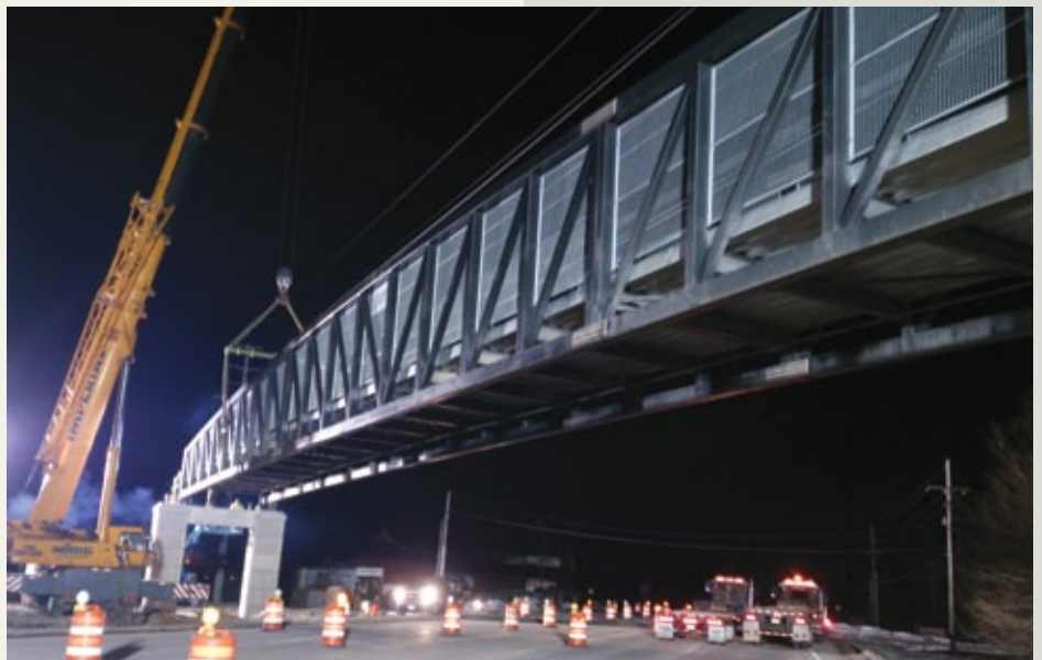
Peoria Park District-Rock Island Greenway new bridge in Peoria, IL
