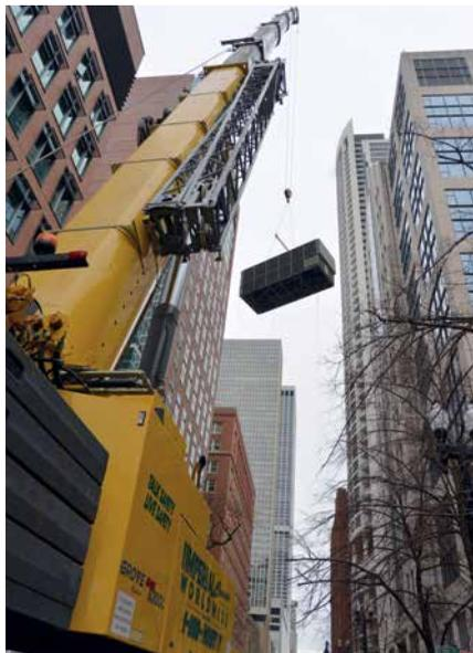
The GMK 6300L was rigged with its full counterweight of 220,000 pounds. Fully rigged the crane was set up at 38-foot wide including the outrigger mats setting up on a 40-foot wide street.
