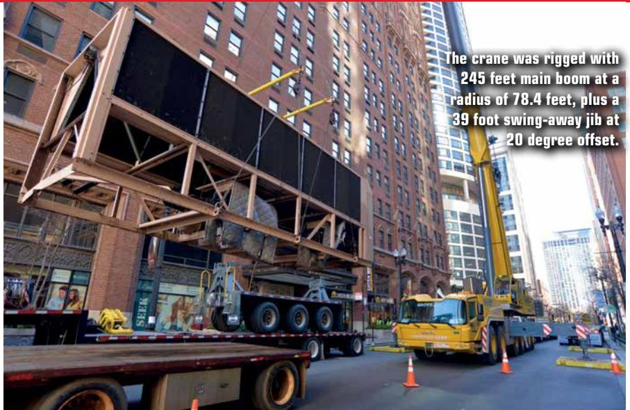
The crane was rigged with 245 feet main boom at a radius of 78.4 feet, plus a 39 foot swing-away jib at 20 degree offset.
